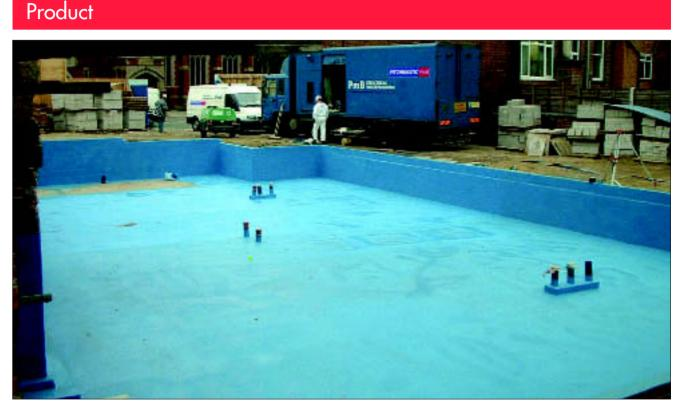
• THIS CERTIFICATE REPLACES CERTIFICATE No 01/3851 AND RELATES TO THE PmB TANKING WATERPROOFING SYSTEM, INCORPORATING A TWO-PART, SPRAY-APPLIED, BLUE-PIGMENTED POLYURETHANE ELASTOMER.
