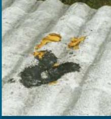
Roof decks encountering high winds can be damaged as a result of high-pressure differentials. When a door or window fails, this pressurization's effect on the roof increases, with dire consequences—the deck (and the roofing membrane) can quite literally blow up. Using SPF on the deck underside could have potentially helped.
