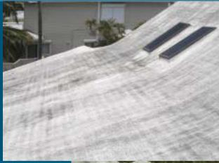
In the summer of 2004, four hurricanes ripped through Florida, causing rampant damage. However, the qualities of spray polyurethane foam (SPF) and other plastic adhesives meant some roofs survived largely unscathed and prevented many materials from becoming missile debris.
